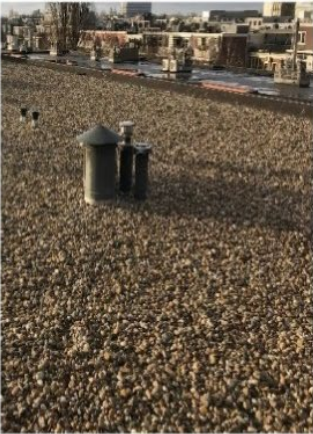
Roof surface with gravel, iButtons have been burried under the gravel
