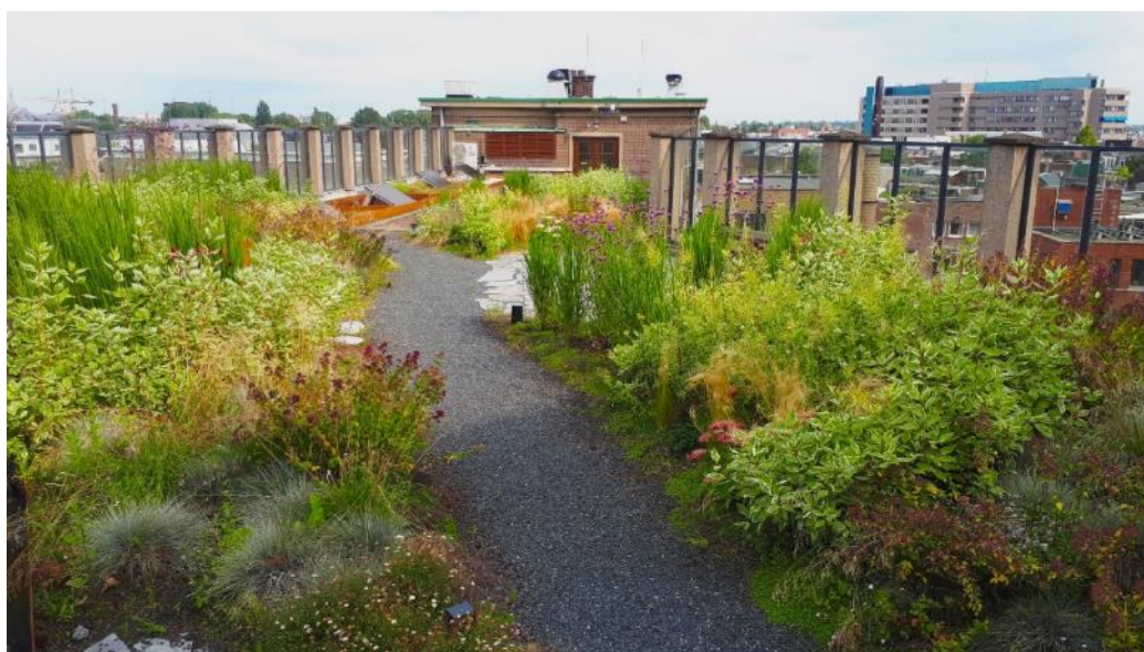
Figure 1 A RESILIO blue-green roof implemented at the Benno Premselahuis (Amsterdam East). The green layer with a mix of different plant species is visible. The blue water retention layer is located underneath the substrate.
