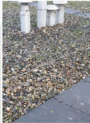
Roof surface with gravel at Oosterparkbuurt, iButtons have been buried under the gravel
