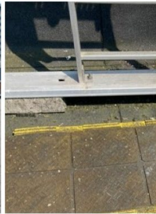
Roof surface with bitumen. iButtons have been placed in the sun and in the shade on the surface
