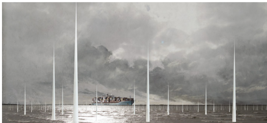
Perforated needles: the deposit is collected and suction-dredged away during low tide.
