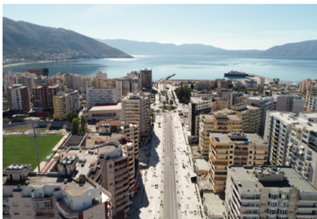
Vlorë Avenue under construction.
