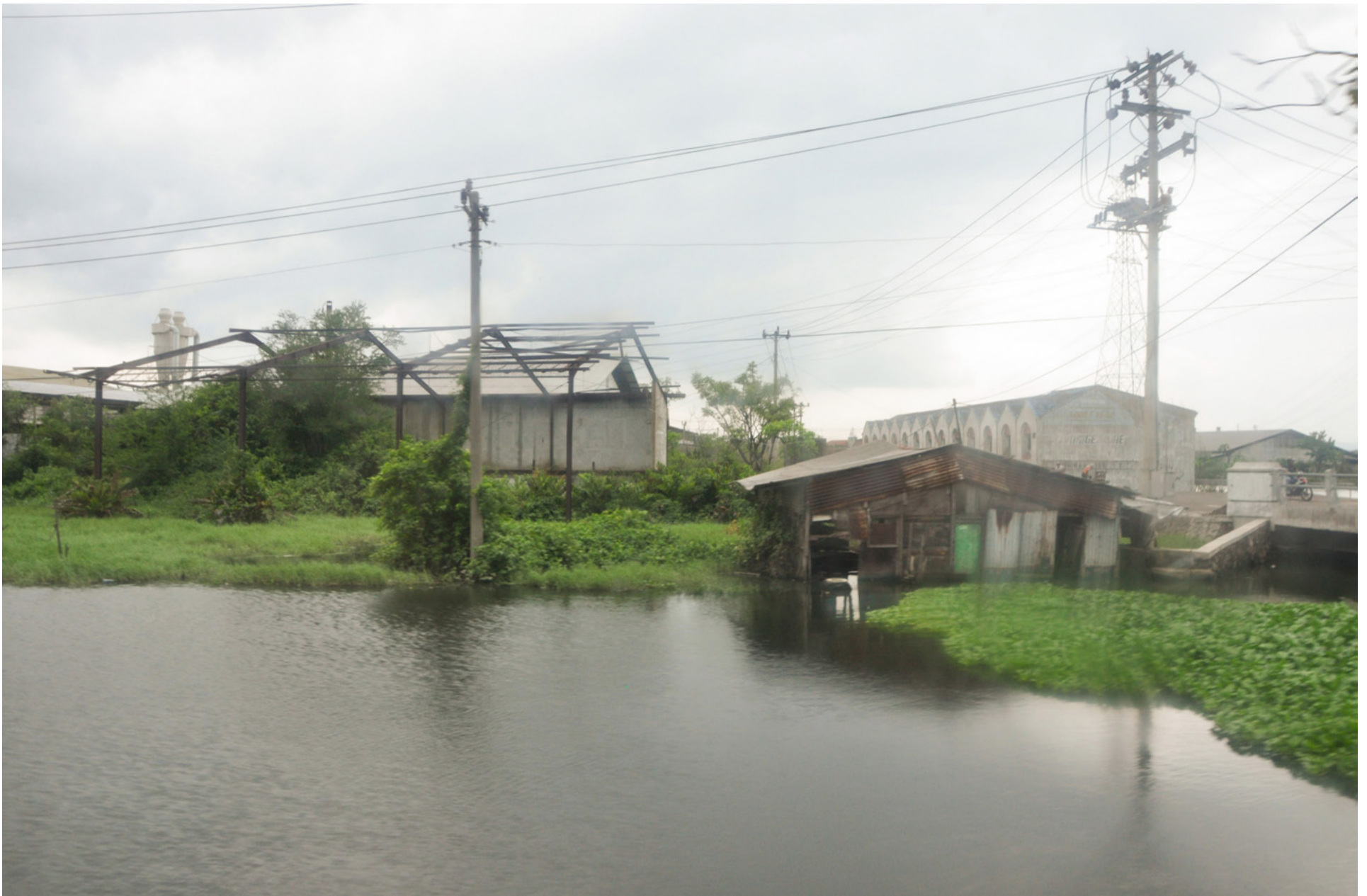
Subsiding industrial buildings on an industrial estate.
