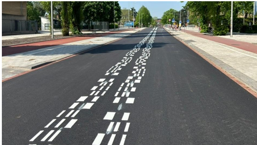
Characteristic wide centre line on GOW30 roads
